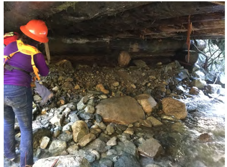
Left Bank Abutment when facing downstream
