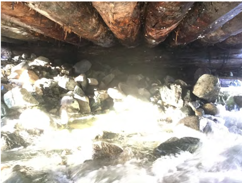
Right Bank Abutment when facing downstream
